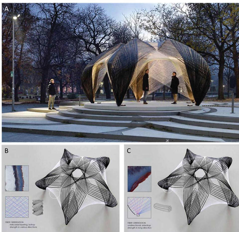
**Figure 20.** (A) The completed ICD/ITKE Research Pavilion, along with architectural designs incorporating (B) a heliocidal structure for isotropic response and (C) unidirectional fibers for anisotropic loading. Reproduced with permission.<sup>[179]</sup> Copyright 2012, ICD-ITKE.
